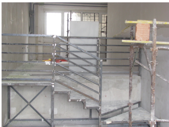
Picture 2. Reconstruction of Urban Permit Center
